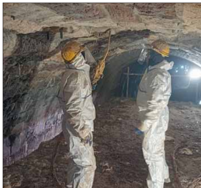
Obr. 7 Reinjektáž v klenbe tunela Fig. 7 Reinjection in the tunnel vault
